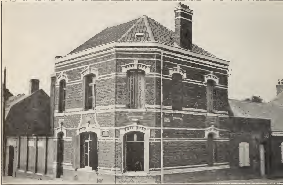
THE NEW "HOME" FOR THE WORK IN RUE CRONSTADT
